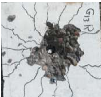
Fig. 11. Crack Patterns ( reference mix )
